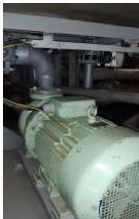
Figure 12: Self-cleaning Filter Pump
