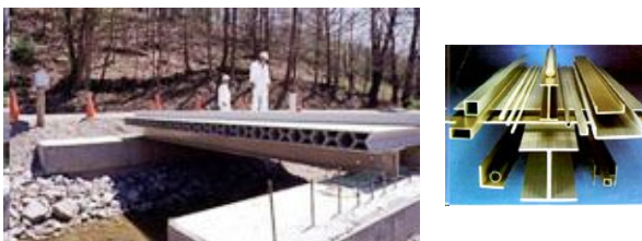
FiberlineBridge, using the pultruded profiles [1]
